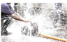
Water pipe cracking leaks
